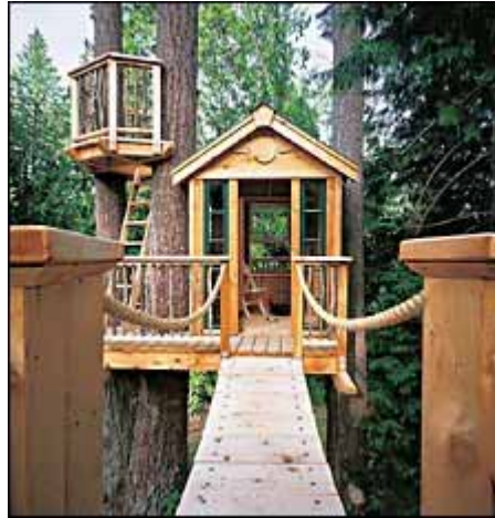
The windows are from building-supply salvage stores, but the Seelys had the glass replaced with tempered panes for safety. Bird watching really means watching out because industrious hummingbirds swoop and buzz visitors.
